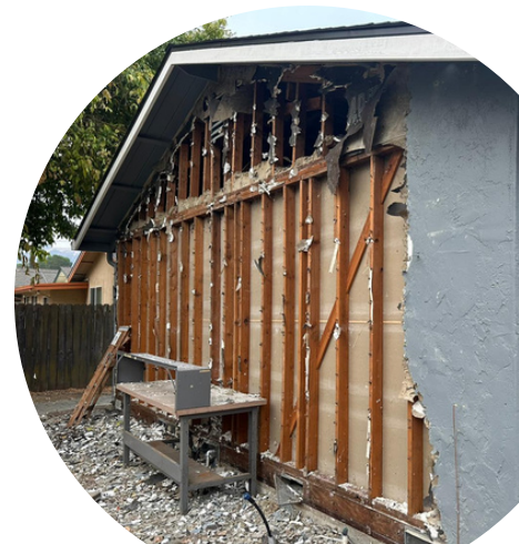
Construction begins at Spring Ave.
